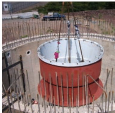
Retube canister liner tubes being installed at the Phase III development area of the Solid Radioactive Waste Management Facility
