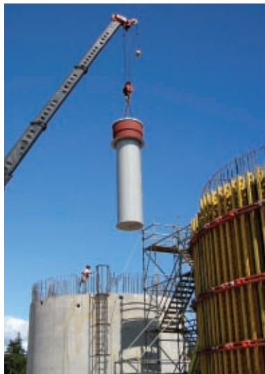
Retube canister liner tubes being installed at the Phase III development area of the Solid Radioactive Waste Management Facility
